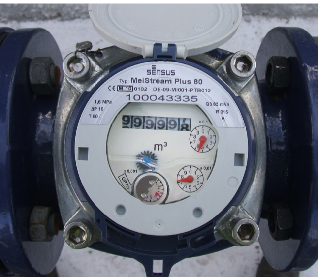
New water meter being installed
