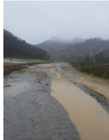
Pictured: Slips at Rawhitiroa Road and Glen Nui Road and flooding on Lakes Road
