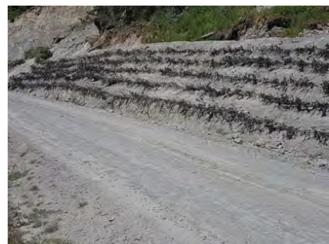
Pictured alongside a completed brush layer wall.
