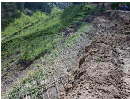
Pictured alongside a completed brush layer wall.
